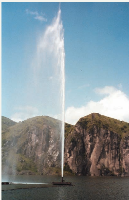
Deep waters in Lake Nyos are pumped to the surface to remove dissolved \text{CO}_2 gas.
